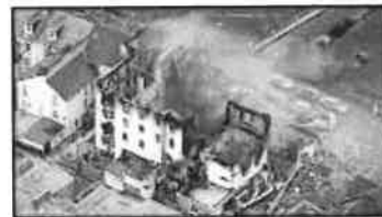
Newquay Hotel – Example where compartmentation failed
